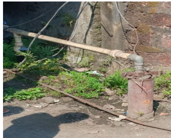
Bore wells without piezometer and water meter in Odisha
