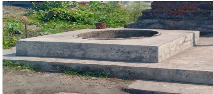
Dug well constructed without permission of CGWA
