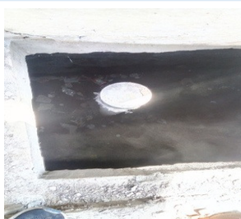
Muddy and water logged RWH structure at Apparel Export Promotion Council, Faridabad
