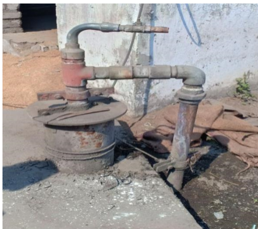
Bore wells without piezometer and water meter in Odisha
